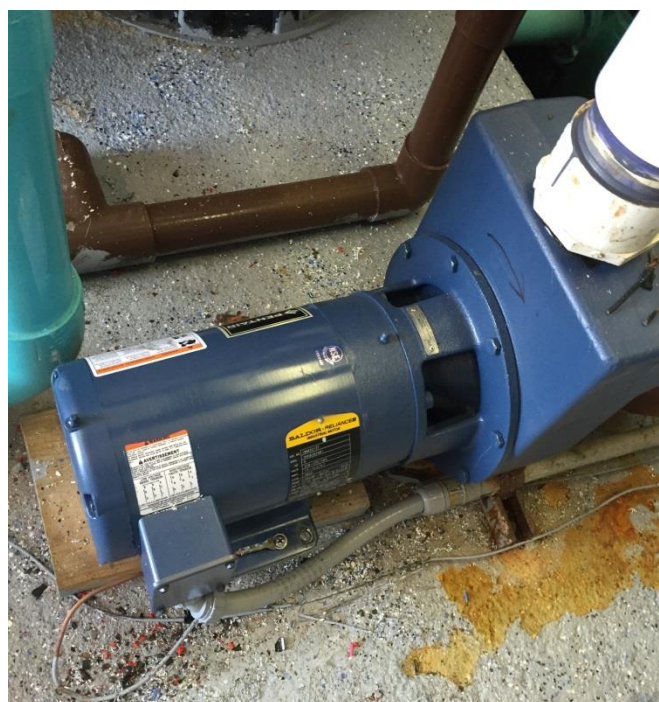
5 hp three phase pump and motor
