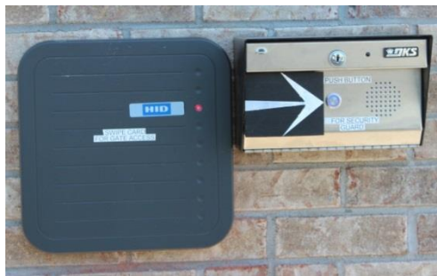
Gate entry system
